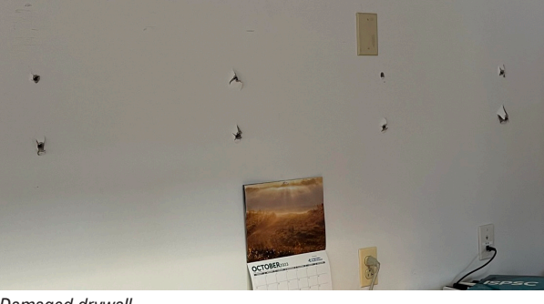
Damaged drywall
