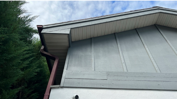
Wood siding & aluminum soffits
