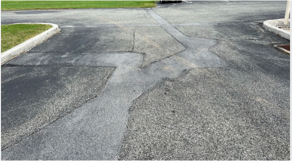
Patched asphalt roadway/parking
