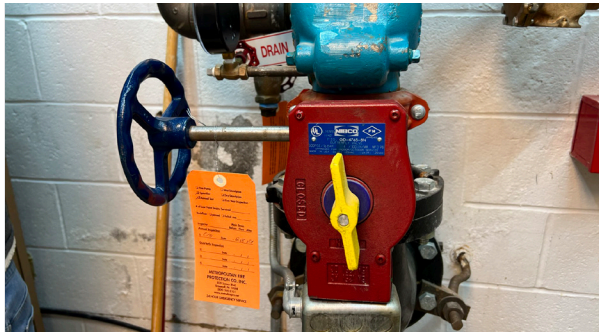
Sprinkler control valve
