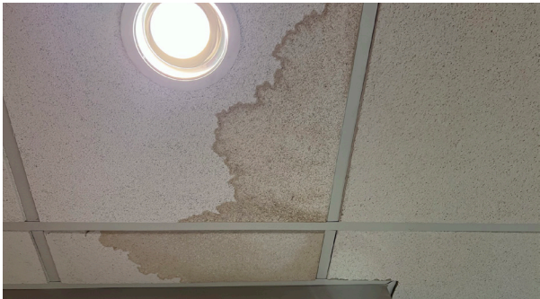
Damaged ceiling tiles
