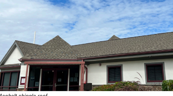
Asphalt shingle roof
